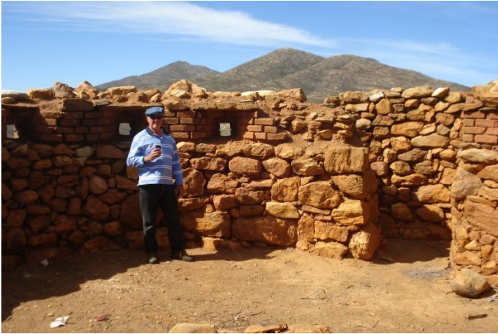
FORT 1 Interior showing loopholes (behind Alwyn) and entrance on right
